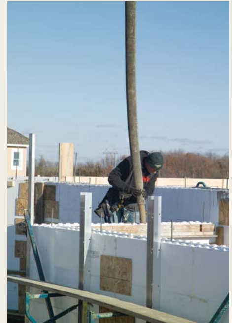
Above and at right: ICFs are hollow foam blocks which are interlocked and stacked to form the shape of the exterior walls of a building or home, reinforced with steel rebar and then filled with concrete.
