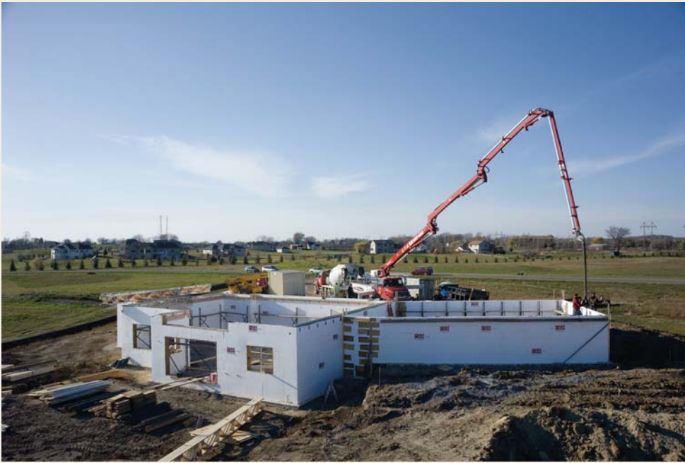
Above and at right: ICFs are hollow foam blocks which are interlocked and stacked to form the shape of the exterior walls of a building or home, reinforced with steel rebar and then filled with concrete.
